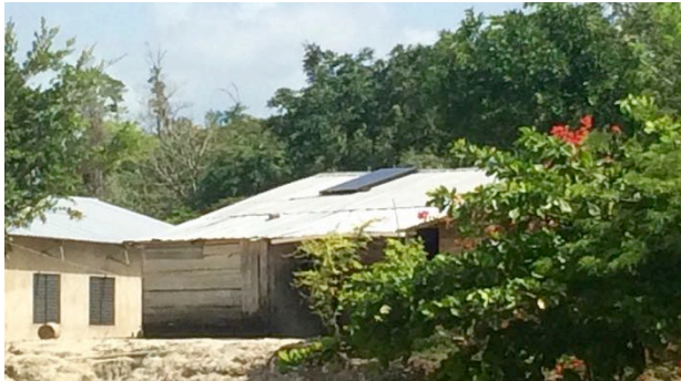
Picture 9: Solar Power System Ex. 3
